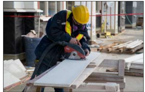
Protected worker cutting fibre-cement board using a circular saw with dust controls
